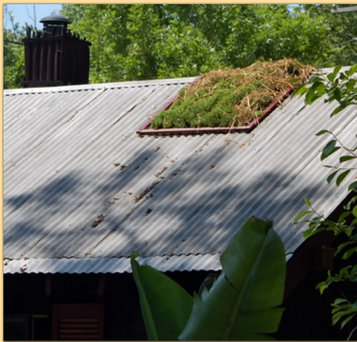
A living roof adds another shade to the already "green" museum building.
